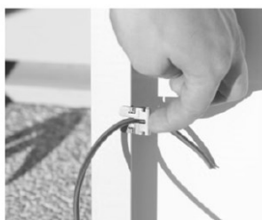
1 Position grounding clip with electrical cable inserted in it and the bottom of the part outside the frame
